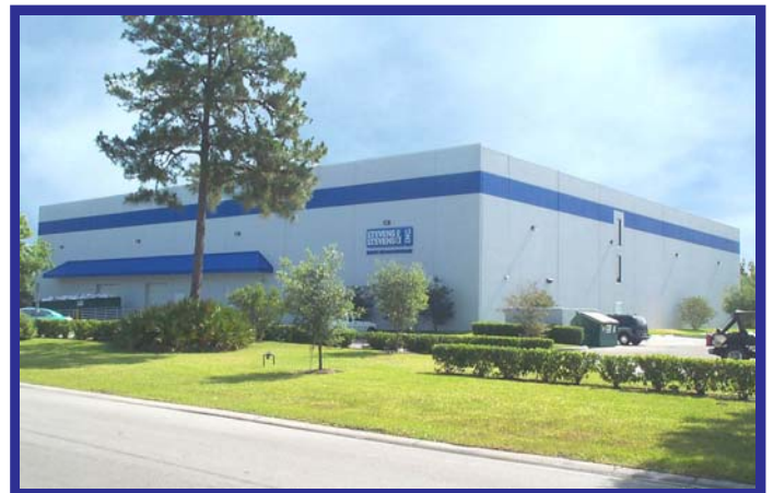
This three story, 30,000 sq. ft., tiltwall structure was designed and constructed by Scherer. It serves as a storage facility for documents and records.
