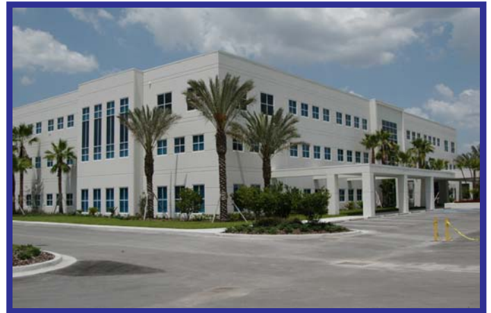
This three story, 100,000 sq. ft. , tiltwall structure is located in Tampa, Florida. It serves as the Florida headquarters for the Salvation Army.
