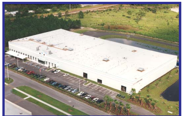
This two story, 80,000 sq. ft. , tiltwall structure is located in Tampa, Florida. It functions as a manufacturing facility for modular office furniture.
